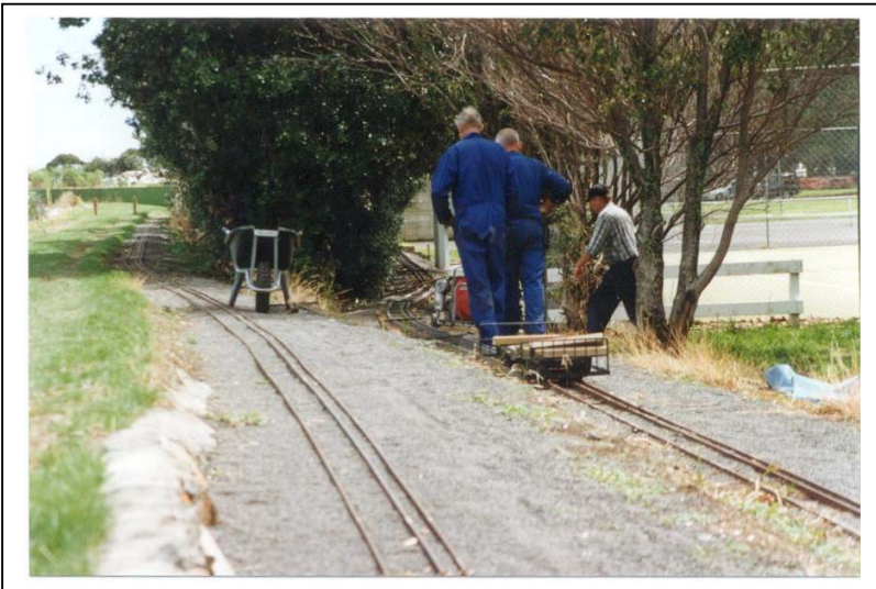
The last few sleepers are laid to join the track.
