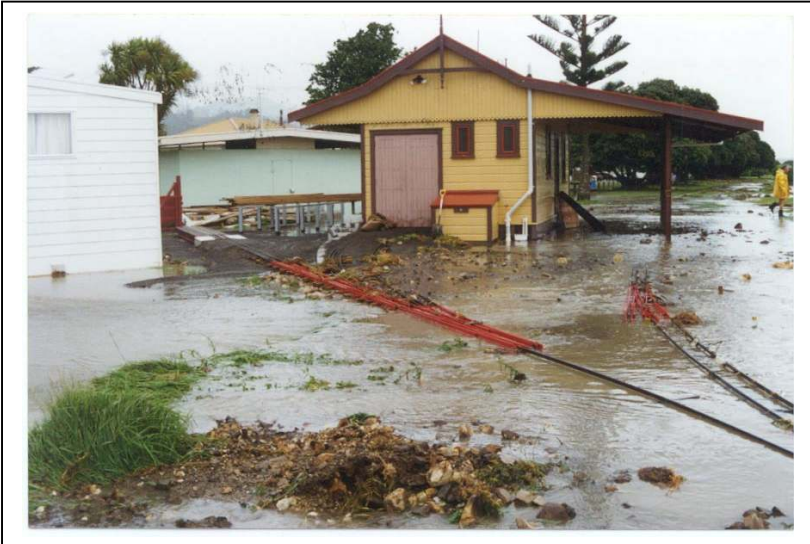
The flooded track after cyclone Drena in January 1997
